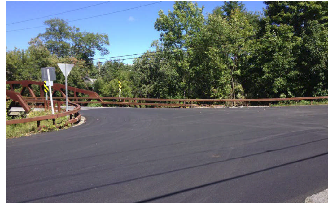
Recently repaved section of River Street near the Judd Bridge Intersection. Note Warren County plans to install new crosswalks and stop signs.
