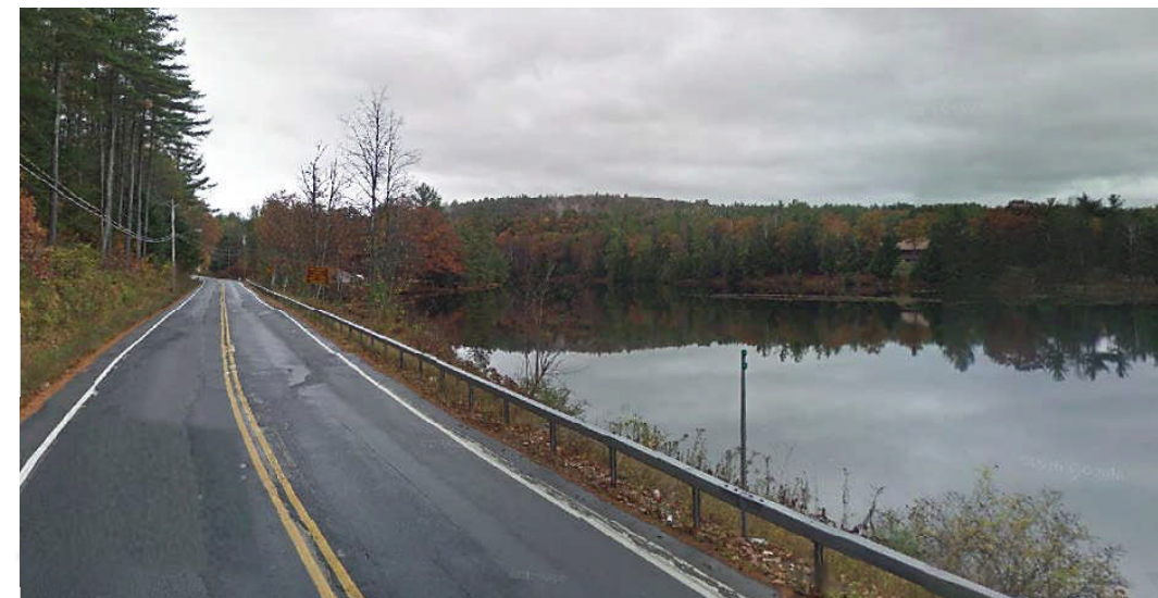
Western portions of the River Street corridor is predominantly defined by a more rural characteristic (courtesy Google Street View)
