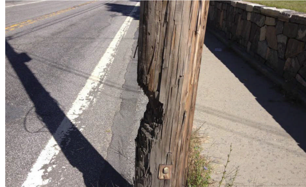
Evidence of vehicle and/or snow plow impacts can be seen on several utility poles within the corridor. Other utility poles are considerably closer to the travel lane.
