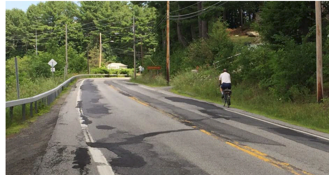
Narrow and poor road shoulder conditions along River Street can deter cycling and can be contribute to a number of safety related concerns
