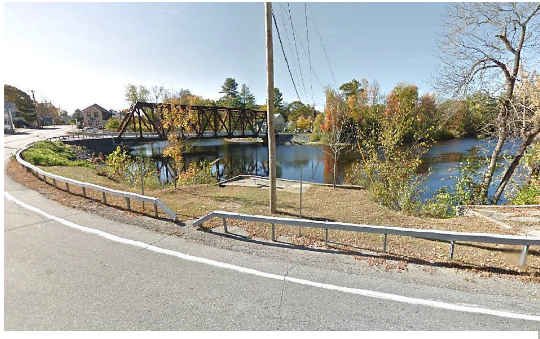
With no sidewalks and only small gap in the guiderail, the small pocket park located opposite the Alden Avenue intersection has limited accessibility (courtesy of Google Street View)
