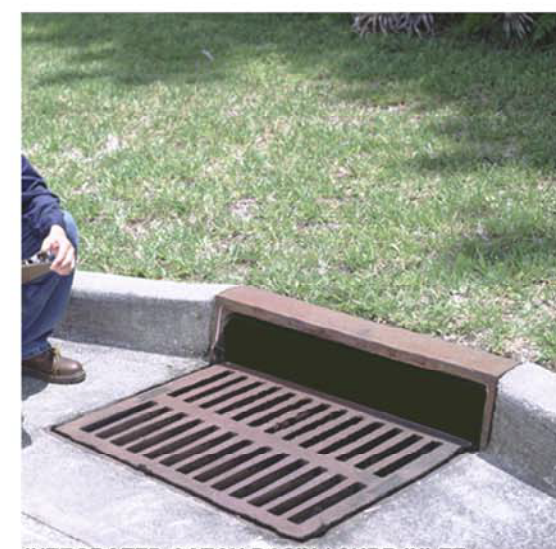
INTEGRATED CATCH BASIN / CURB INLET
